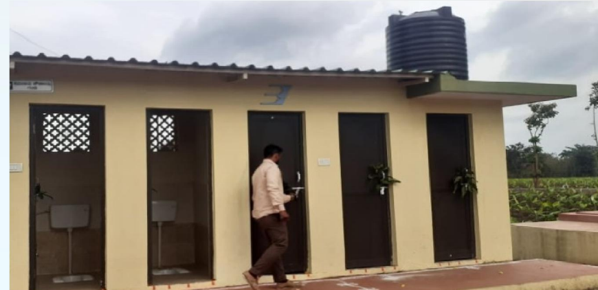
Community Toilets for Tribal community at H.D. Kote, Mysore
