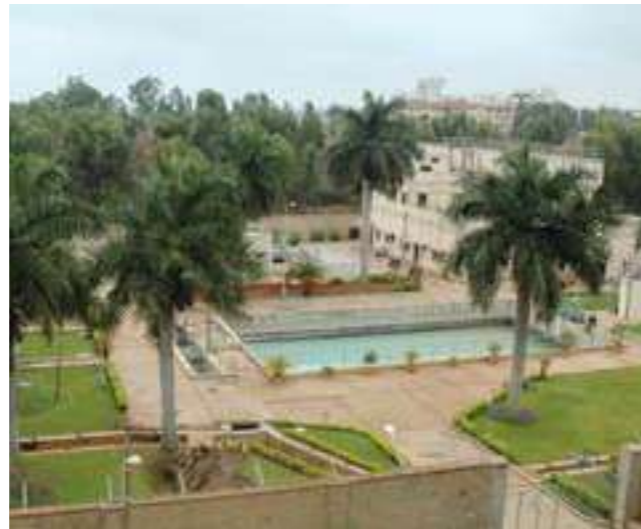
Centralised Effluent Treatment Plant at BEL's Bangalore Complex.
