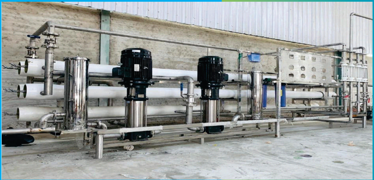
Reverse Osmosis (RO) Plant Equipment to be supplied by BELOP
