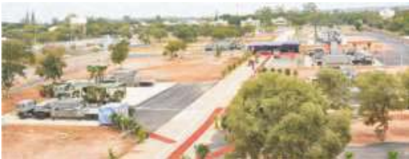
Missile System Integration Facility State-of-the-art facility for testing & integration of various sub-systems of Missile Systems
